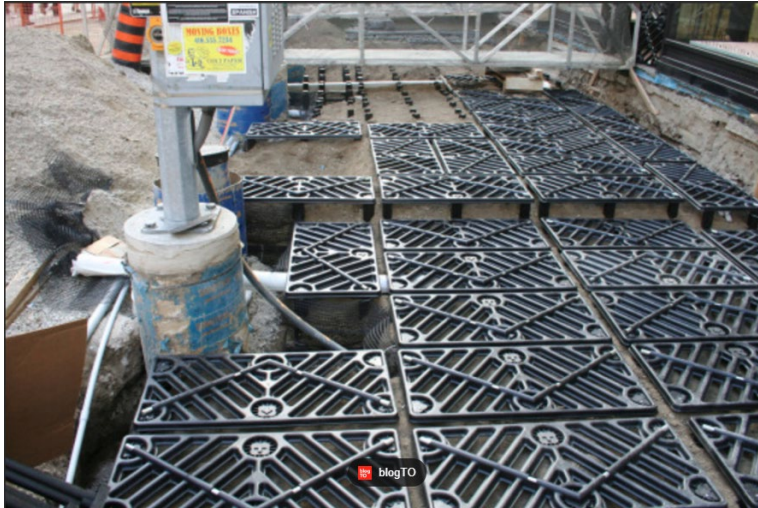
Silva Cells being installed in Toronto, Canada. Web image.
